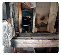
**Image above:** Fire Basement Car Park: Fire spread to the upper floors of the building due to: Poor fire-stopping of penetrations in the concrete slab between the basement car park and the upper floors
