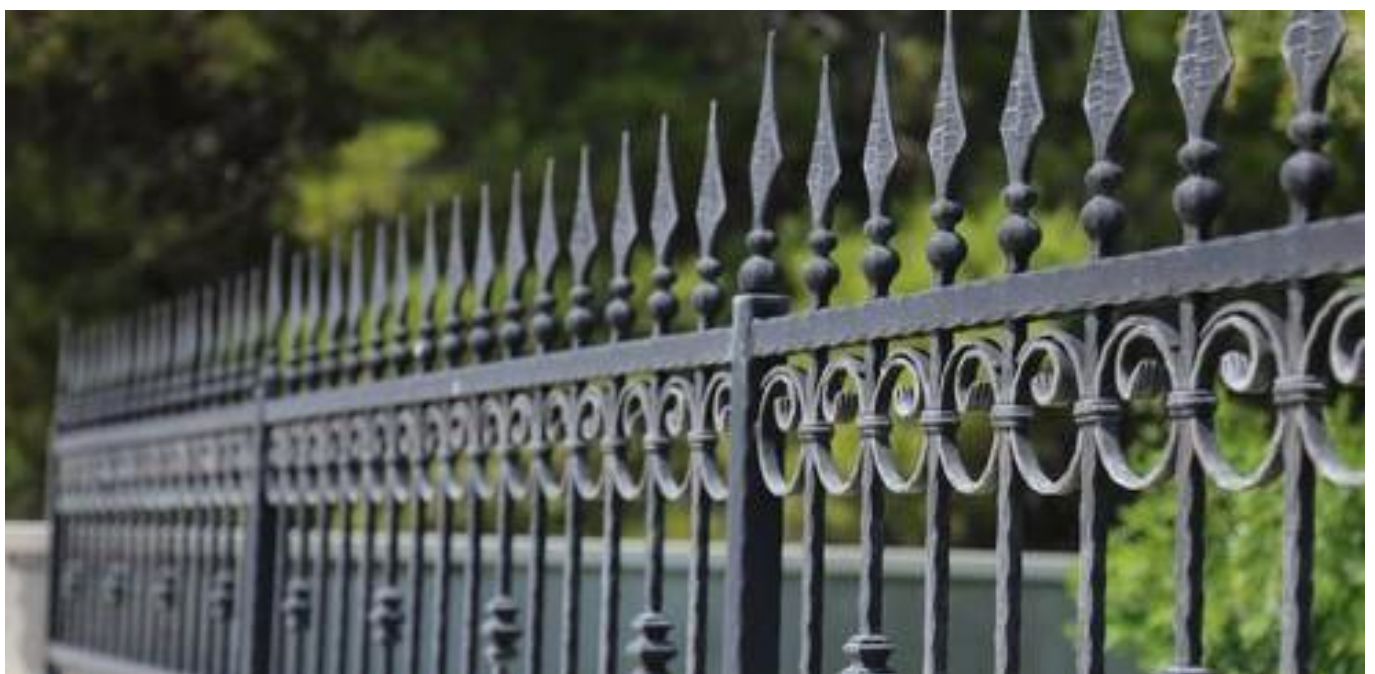
Typical boundary fencing
