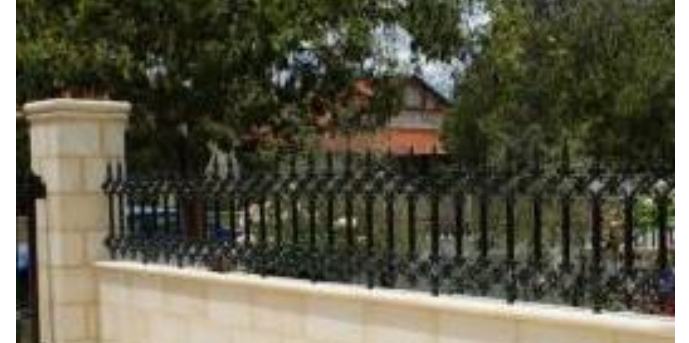
Typical boundary fencing
