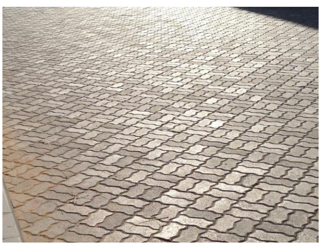
Paving on driveways
