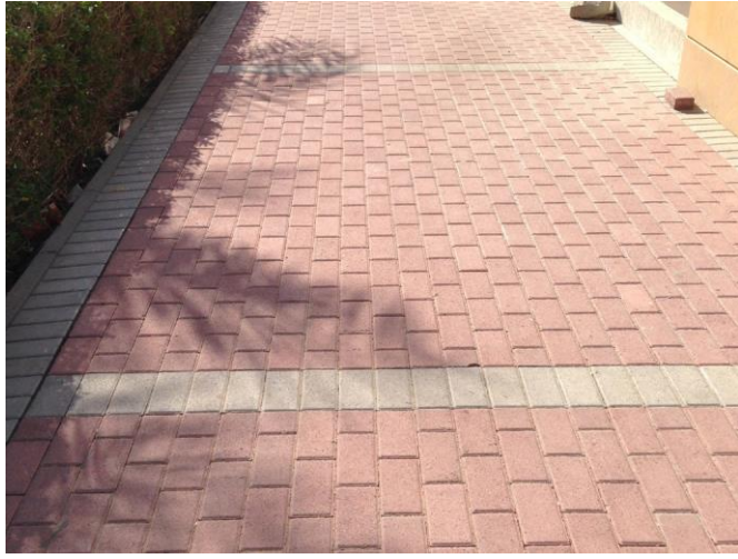
Paving on sidewalks
