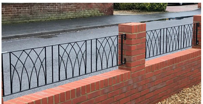
Typical boundary fencing
