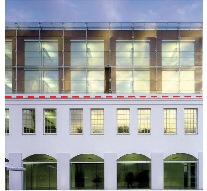
Distinguished top of building design, in harmony with the building components
