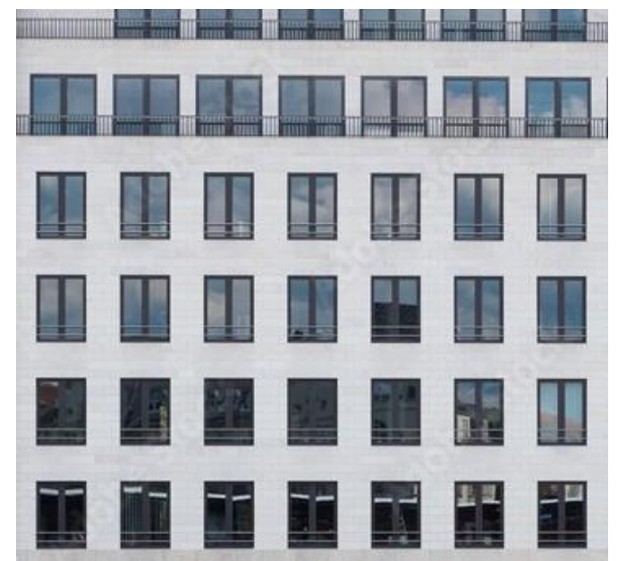
Symmetry & composition - horizontal & vertical alignment. Framed windows
