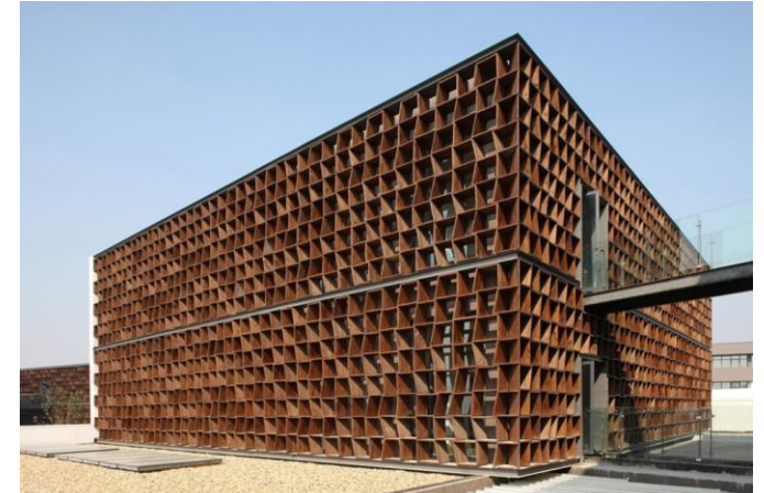
Enclosing utility building in a structure
