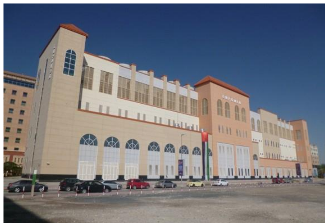
Various samples of district cooling plants where the façade design is in compliance with its development architectural theme
