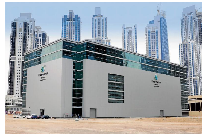
Covering façades should incorporate different depths, materials, colours and lighting. In addition, Landscaping is encouraged as a complimentary aspect to the camouflaging process
