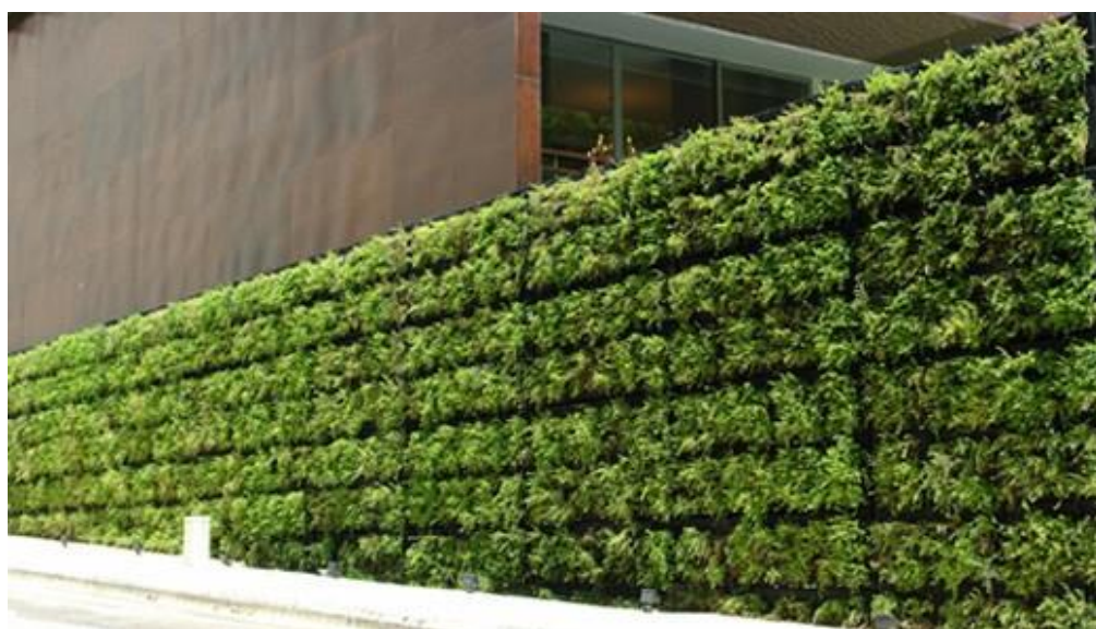
Living walls can be created as individual pieces or in a modular fashion to allow for easy mounting to different surfaces
