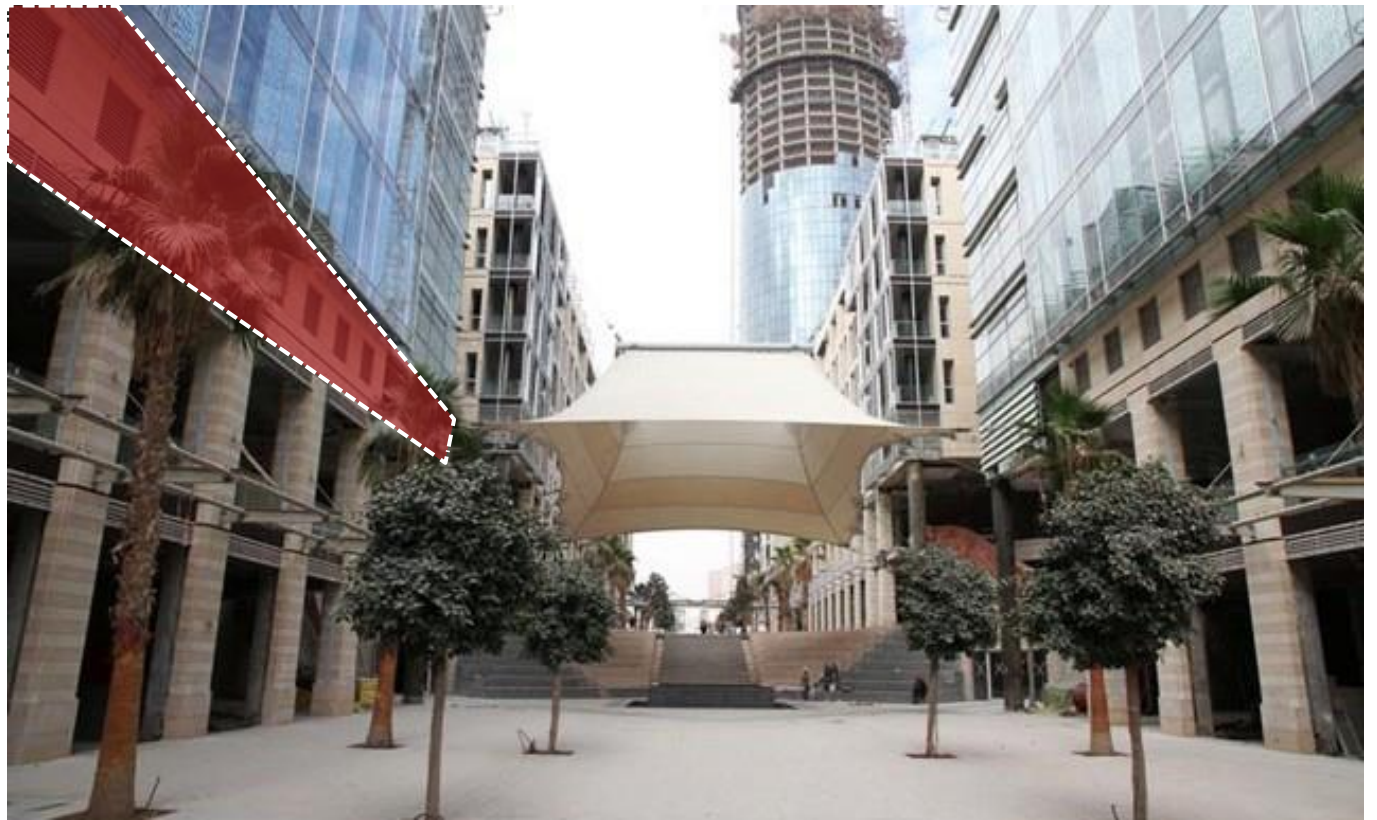
Parking within the podium to be screened. Openings to follow the building grid
