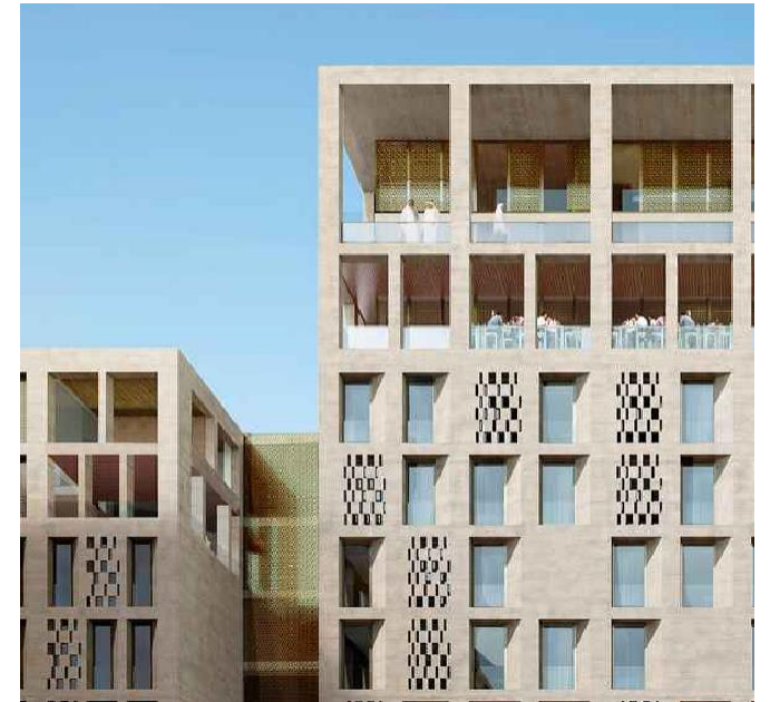
Recessed windows to add depth to the façade; perforated screen to provide shading and privacy
