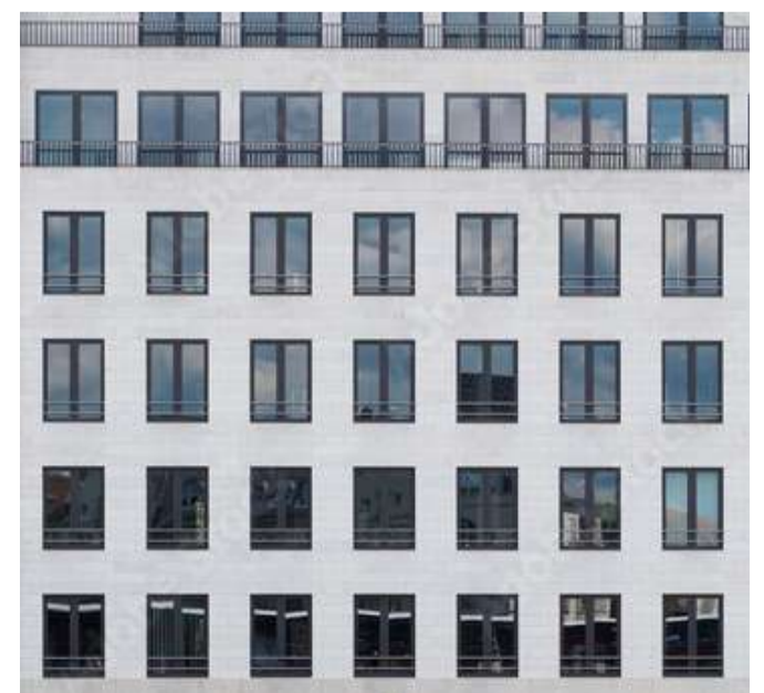
Symmetry & composition - horizontal & vertical alignment. Framed windows
