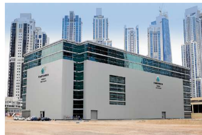
Covering façades should incorporate different depths, materials, colours and lighting. In addition, Landscaping is encouraged as a complimentary aspect to the camouflaging process
