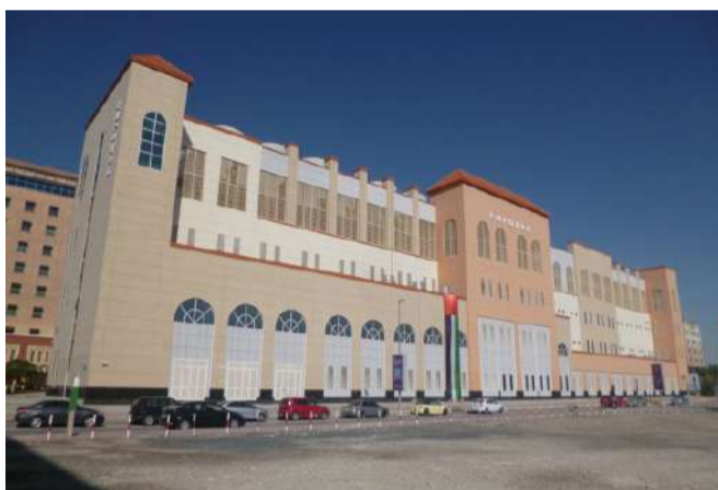
Various samples of district cooling plants where the façade design is in compliance with its development architectural theme
