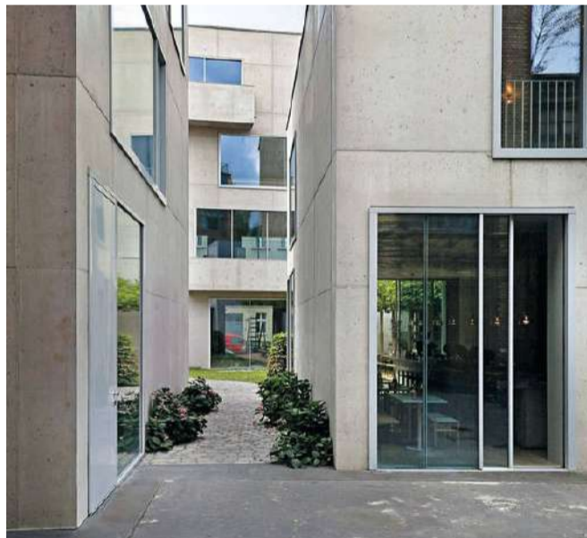
Concrete panels with regular joints
