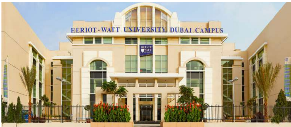
Visible entrance, drop off and pick up area
