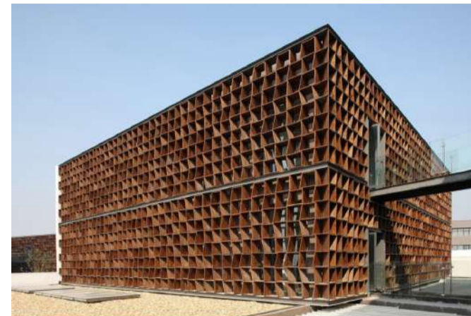
Enclosing utility building in a structure
