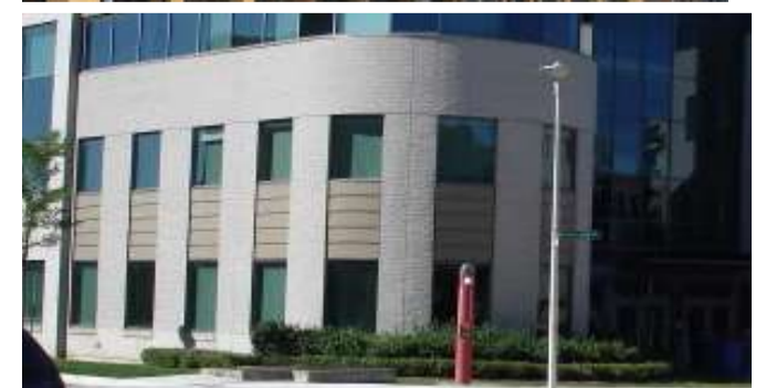
Various façades materials and colors varying between terracotta and Gray as primary colors
